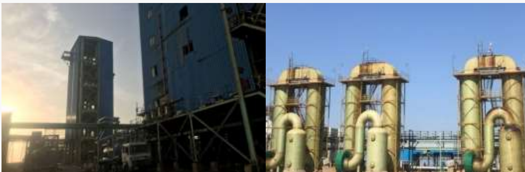
Exhibit 21: ACIL Bromine Production Plant Facility
